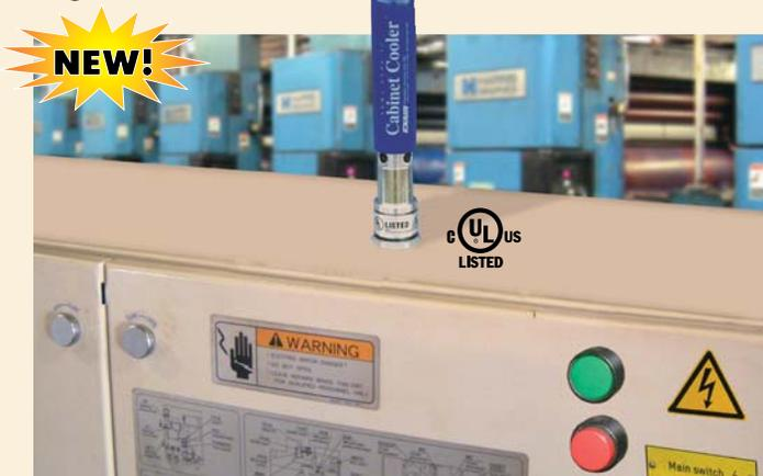
**Cabinet Coolers eliminate unexpected shutdowns by keeping the enclosure cool with 20°F air.**
