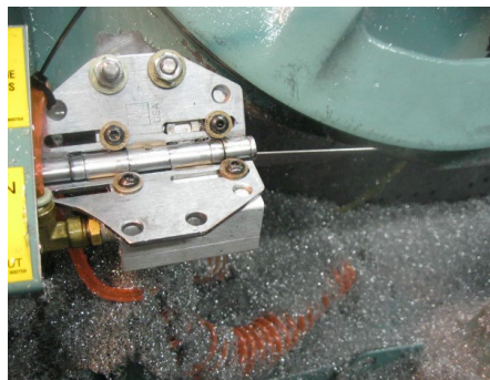
...as well as the drive pulleys and bearings.
